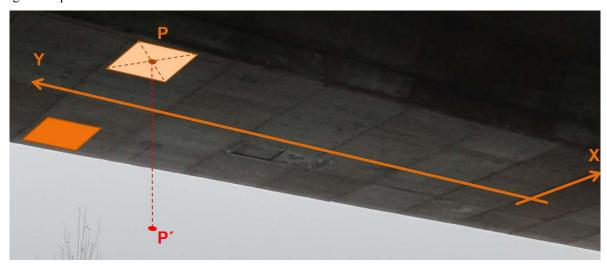
Figure 4: Determination of the height of measured points
