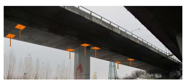
Figure 3: Vertical displacement determination of part of the Harbor Bridge in Bratislava Orthogonal regression is calculated from the general equation of plane:
